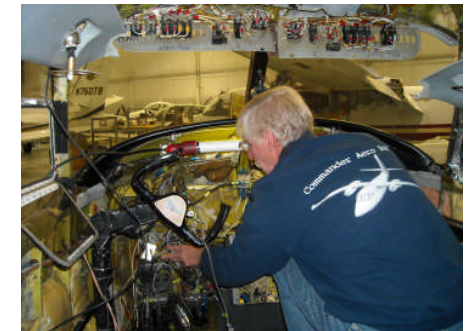
Jack Musgrave in the early stages of providing a complete new panel for N6172X that includes Garmin upgrades and eliminates a mass of extraneous wiring.
