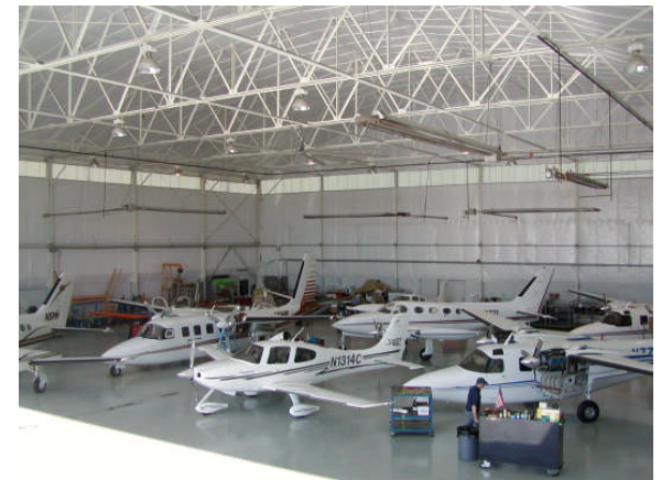
Commander Aero hangar
